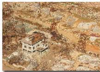
This photo clearly shows the concrete post and beam construction that supports the 3,000 sq ft structure. (Photo courtesy of John Fleck)
